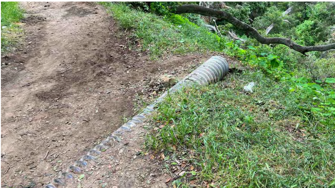
Photo 14. Culvert drainage observed April 28, 2023.
