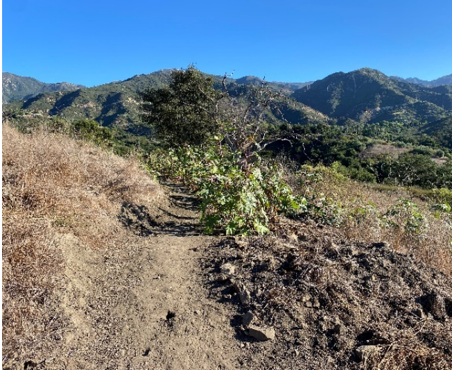
Work Area 2 Before
