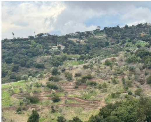
Work Area 4 After
