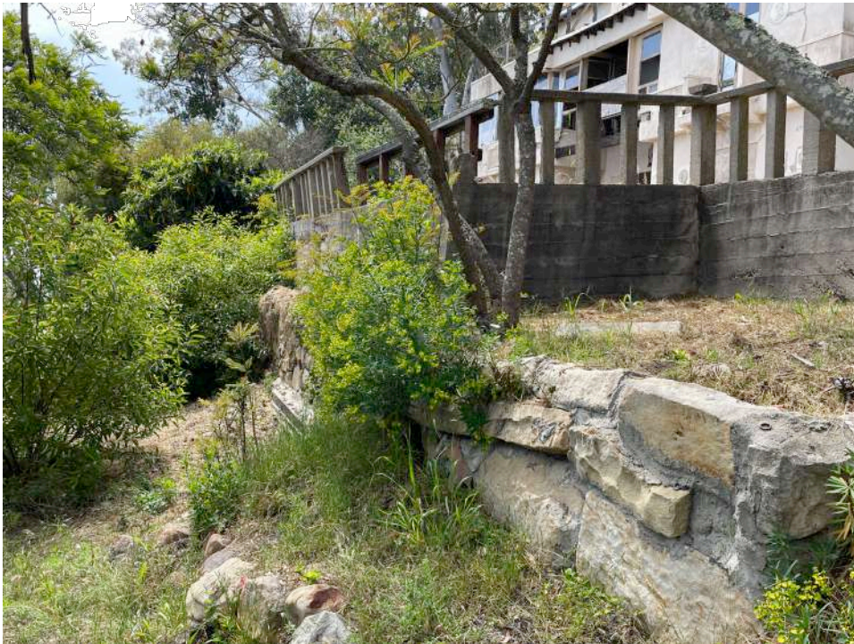
Photo 5: View from SE, (E) retaining walls
