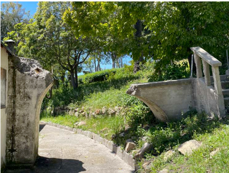
Photo 10: View from E, remnants of arched bridge
