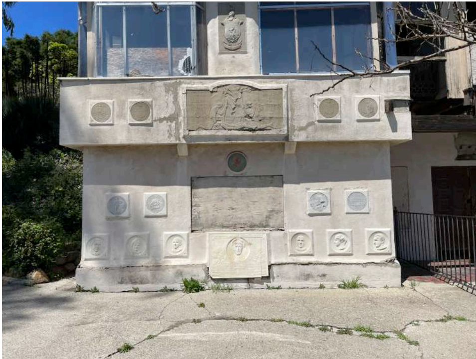
Photo 7: View from S, Franceschi House facade
