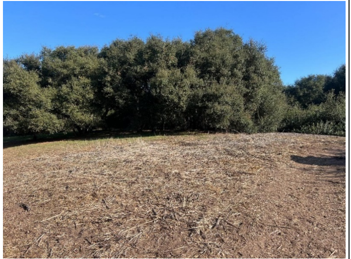
Work Area 20 After
