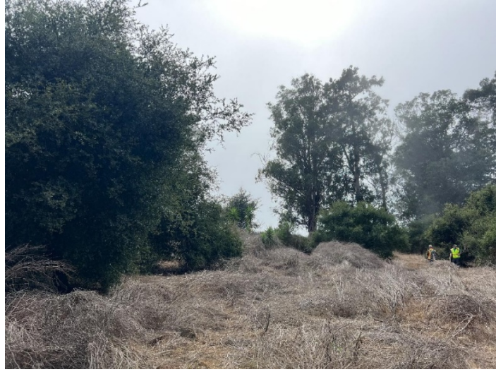
Work Area 6 Before
