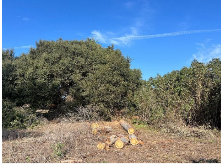
Work Area 40 After
