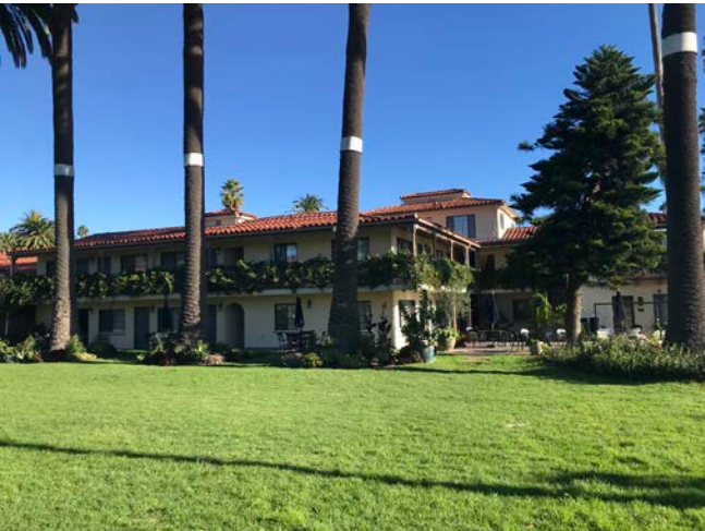
3. View looking northeast at Hotel Milo edge treatment
