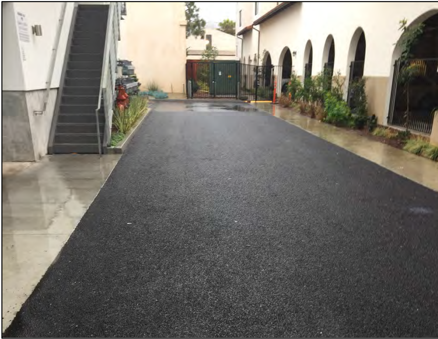
FIGURE 2-8: Permeable Asphalt in Santa Barbara
