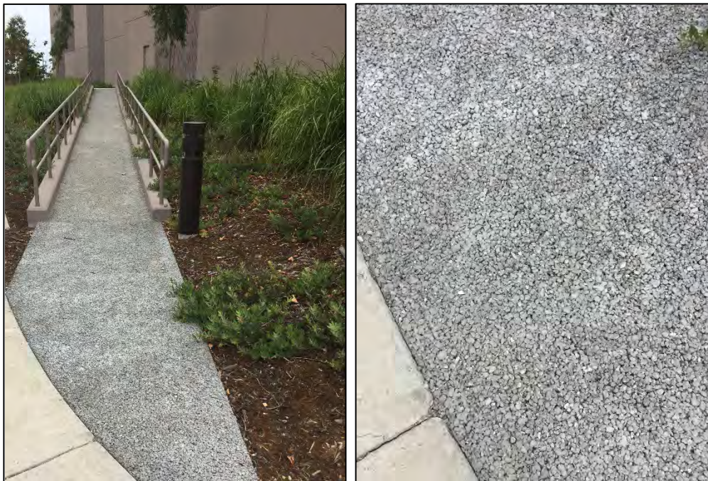
FIGURE 2-9: Permeable Concrete in Goleta
