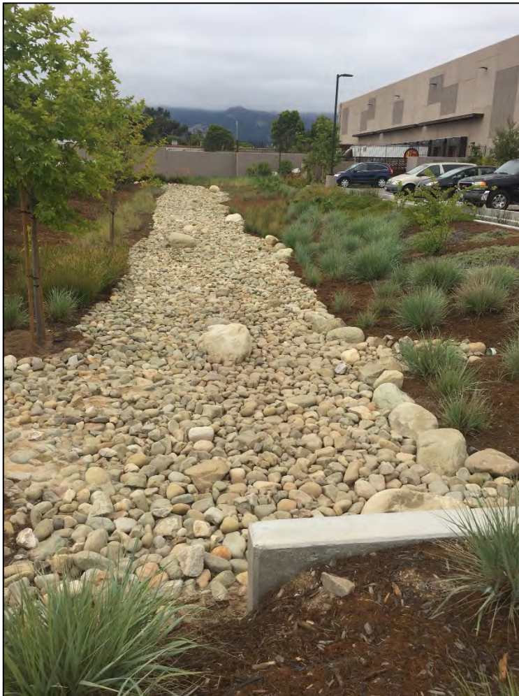
FIGURE 6-27: Dry Extended Detention Basin in Goleta
