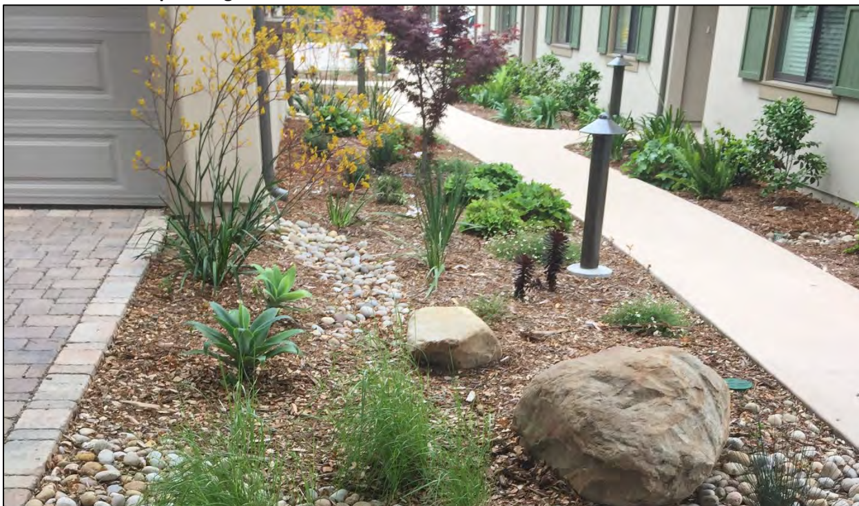
FIGURE 2-2: Flow Spreading in Santa Barbara
