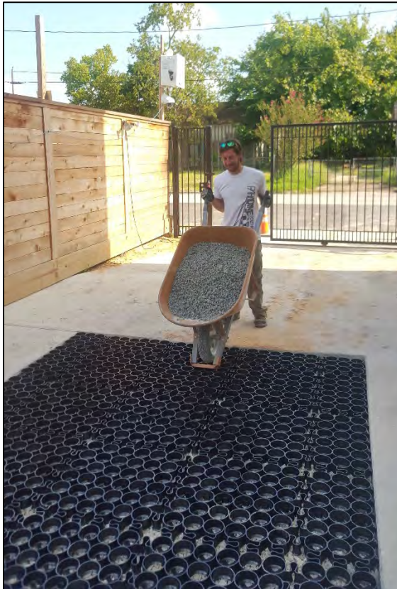
FIGURE 2-12: Gravelpave Multi-Family Residential Driveway
