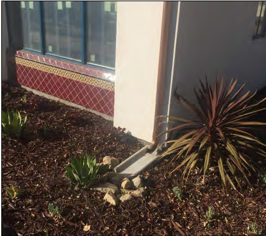
FIGURE 2-1: Disconnected Downspout in Santa Barbara
