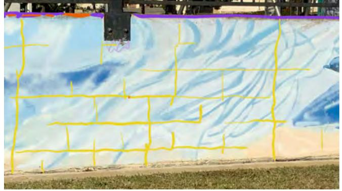
Figure 2. Example of the extensive cracking (drawn in yellow) in the shape of the CMUs found in *Dolphins* and *Codex Cospi*. This type and extent of cracking is what would mak
