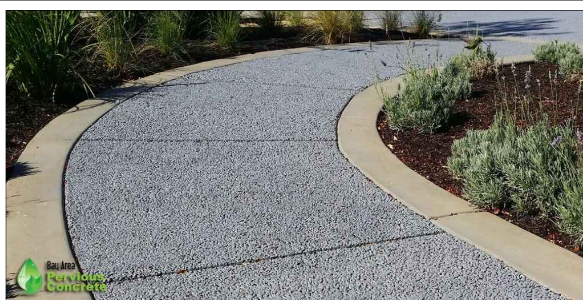
PERMEABLE PAVING AND CURB
